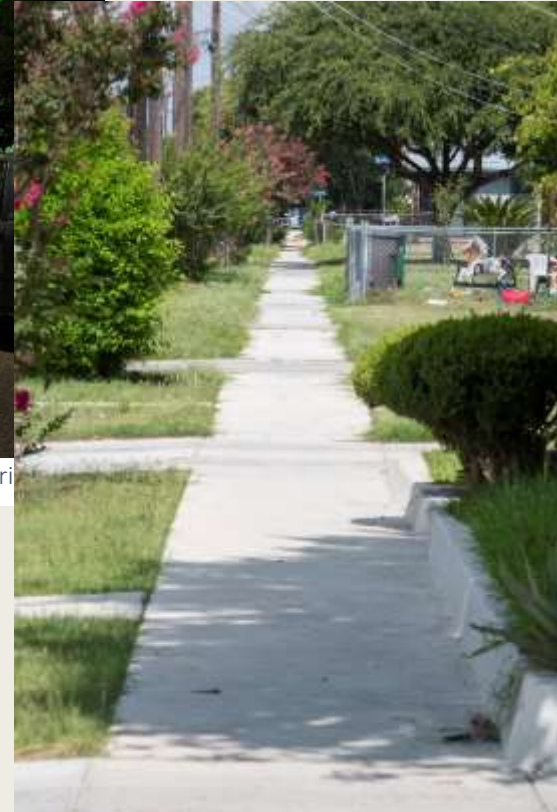
New sidewalk along Burleson St.
