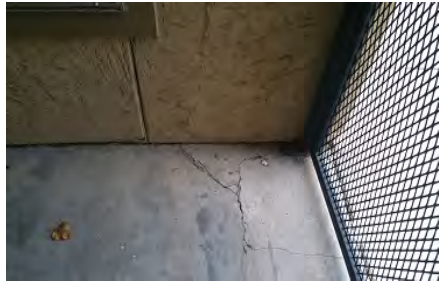
Photo 2 – Walkway Cracks near SE Community Exit
