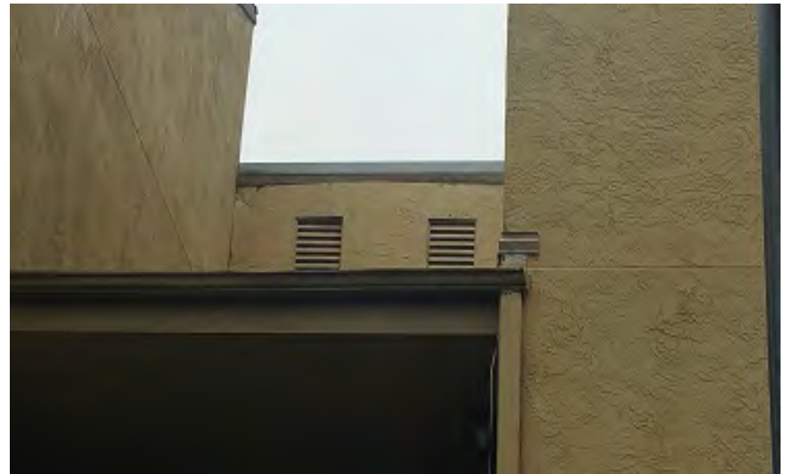
Photo 70 – 3 rd Floor Deteriorated Walkway Canopy Façade between North and East Buildings
