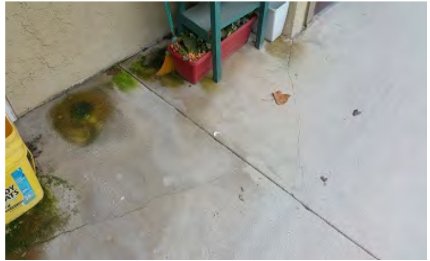
Photo 43 – 3 rd Floor: Walkway Crack
