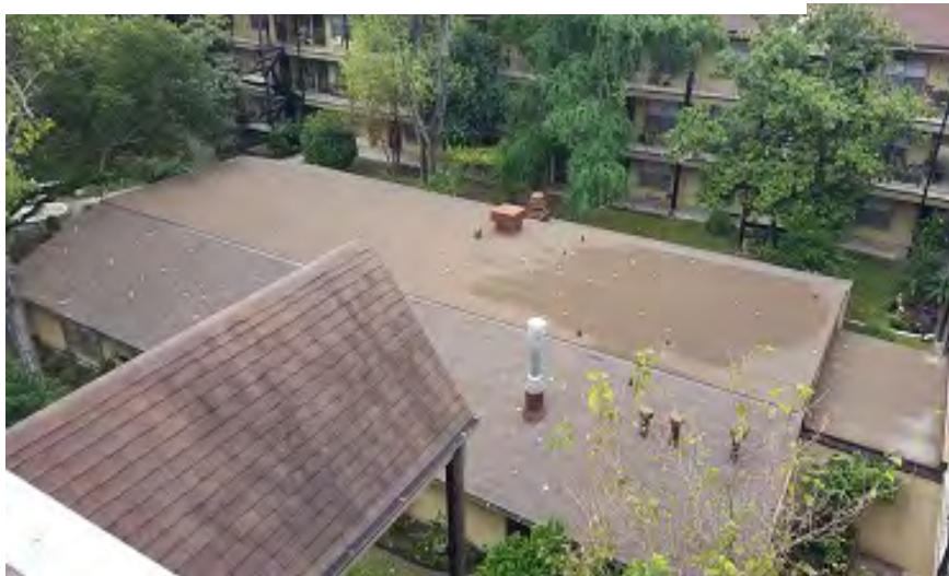
Photo 95 – Community Building Roof (Looking West)
