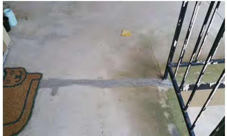
Photo 39 – 3 rd Floor: Walkway Crack
