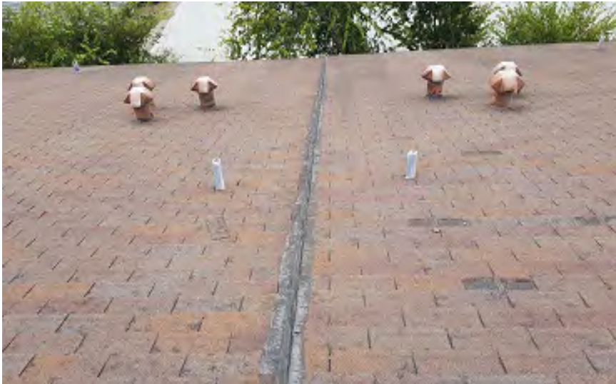
Photo 89 – West Building showing Deteriorated Northern Roof Expansion Joint
