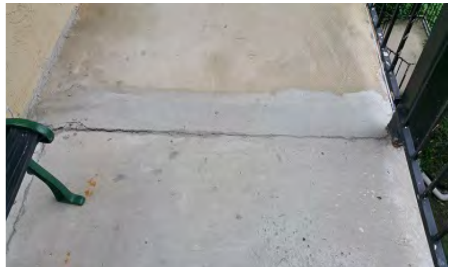
Photo 45 – 3 rd Floor: Walkway Crack
