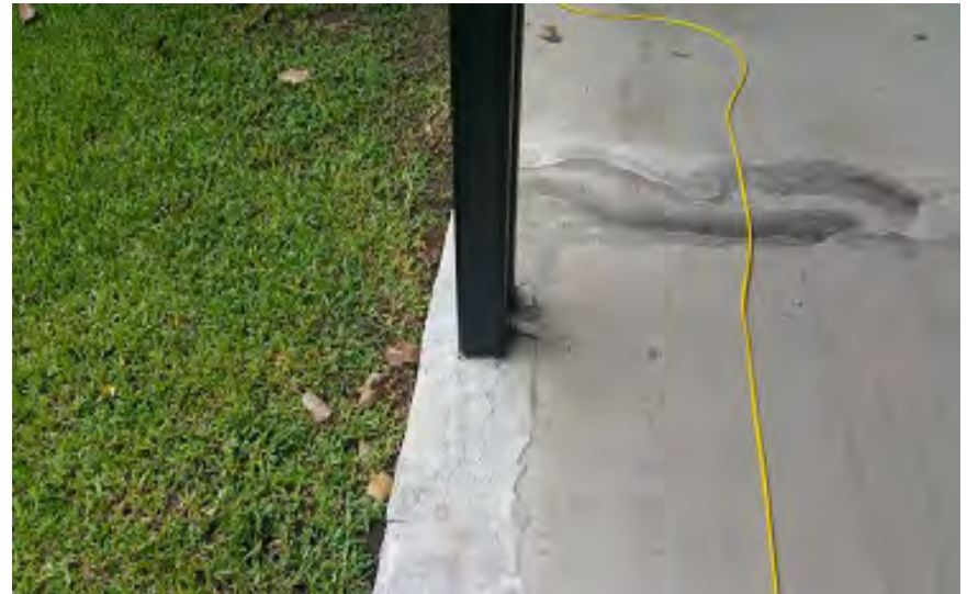
Photo 18 –Walkway Crack near Unit 107
