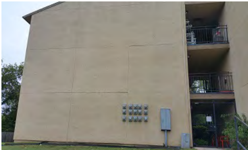
Photo 54 – West Building: South Façade Joint Separation
