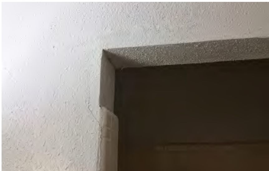
Photo 9 – Unit 113: Cracks Shower Corner
