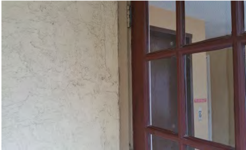
Photo 34 – 2 nd Floor: Wall Crack near Elevator Lobby
