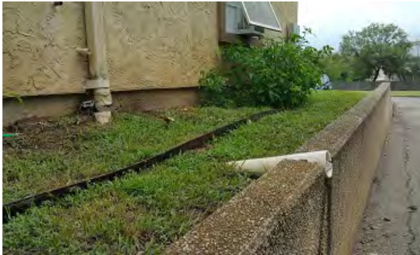
Photo 52 – West Building: Improper Drainage (Looking South)
