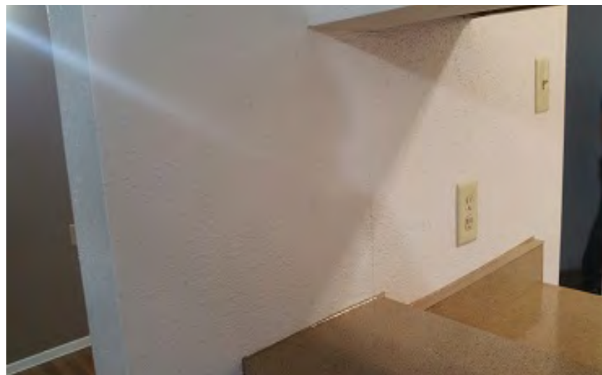
Photo 12 – Unit 112: Crack near Kitchen Counter
