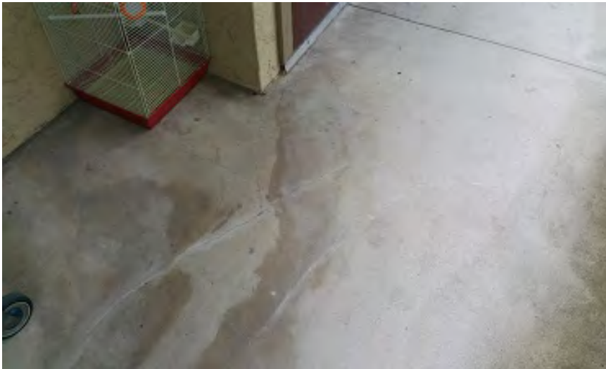
Photo 32 – 2 nd Floor: Walkway Crack
