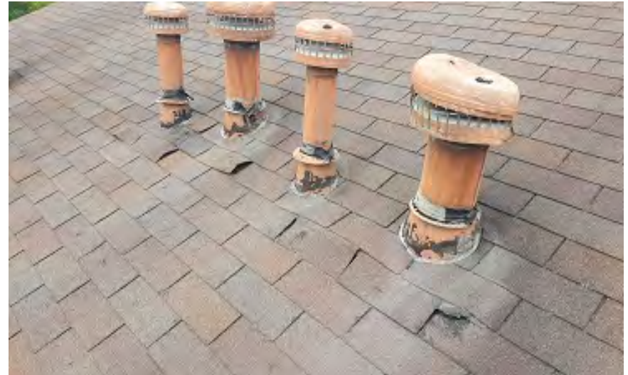
Photo 80 – East Building: Deteriorated Flashing and Roofing at Vent Penetrations
