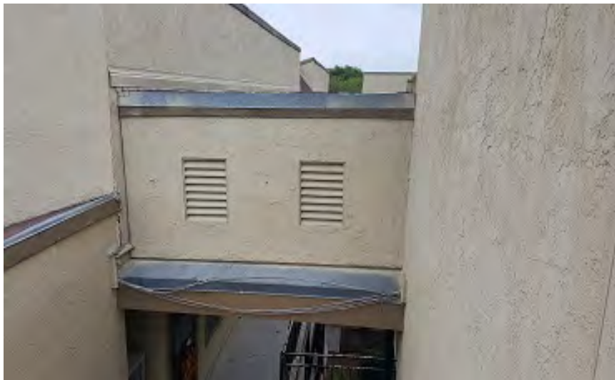
Photo 83 – Walkway Canopy Connector between North and West Buildings showing Deteriorated Conditions
