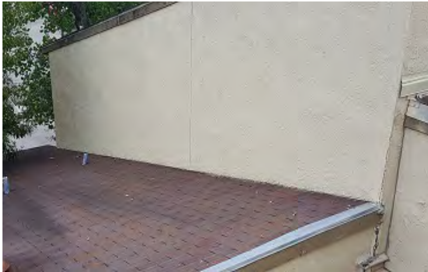
Photo 85 – North Building Roof: West End showing Facade Cracks
