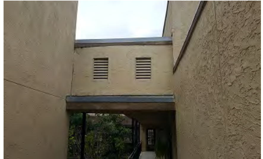
Photo 94 – Walkway Canopy Connector between North and East Buildings showing Deteriorated Conditions
