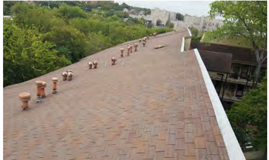
Photo 76 – East Building Roof showing Deteriorated Vents, Penetrations, and Flashings (Looking South)
