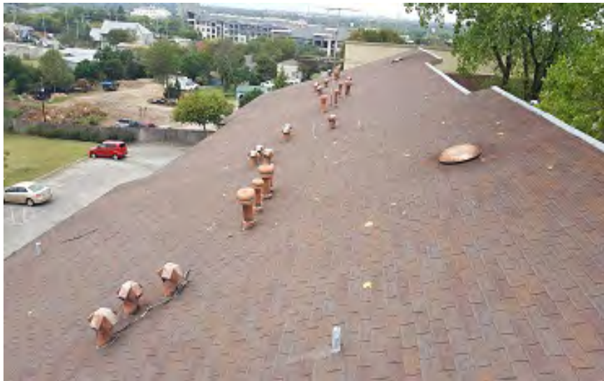
Photo 81 – South Building Roof showing Deteriorated Vents, Penetrations, and Flashings (Looking West)
