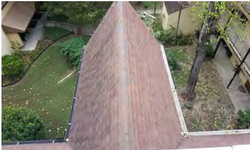
Photo 87 – West Building: Southern Stairway Canopy Roof showing hail Damage (Looking East)
