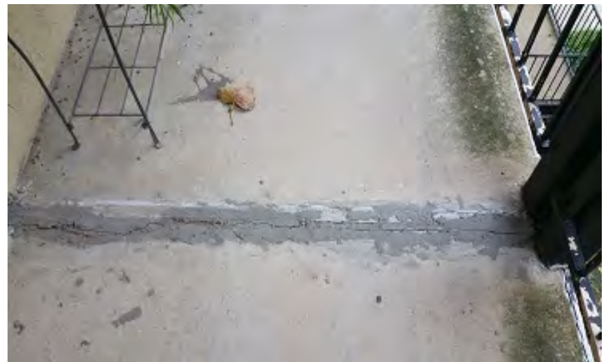
Photo 41 – 3 rd Floor: Walkway Crack
