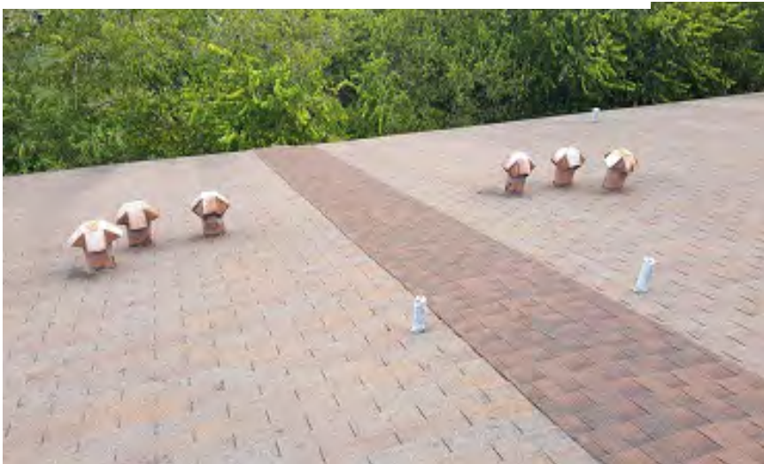
Photo 75 – East Building: Northern Roof Expansion Joint Improperly Covered with a Shingle Patch
