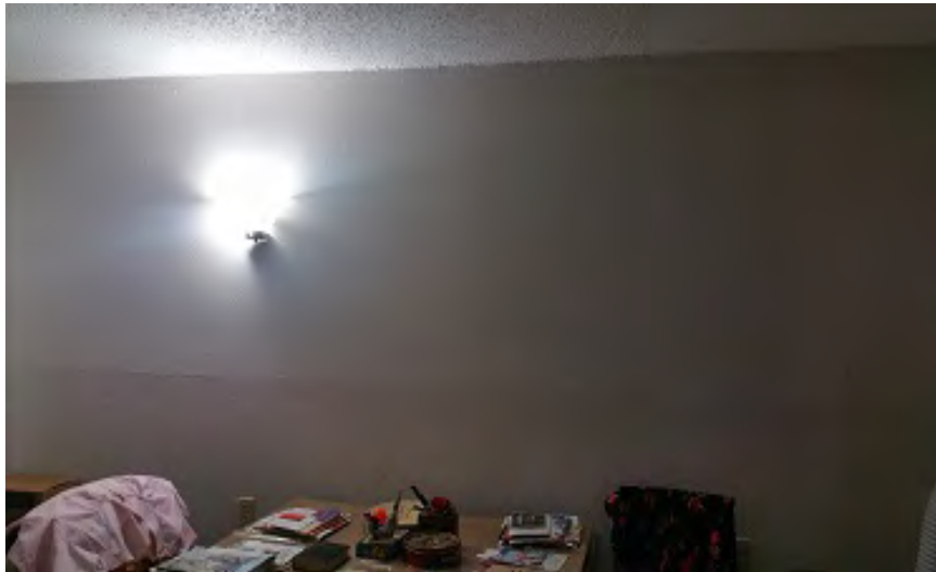
Photo 21 – Unit 103: Crack in Living Room
