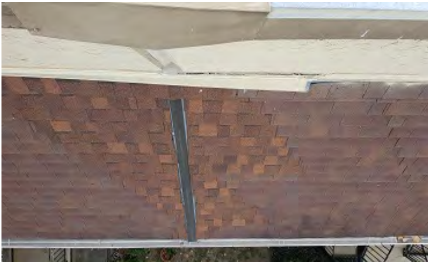
Photo 91 – West Building: Northern Deteriorated Expansion Joint at Walkway Canopy Roof
