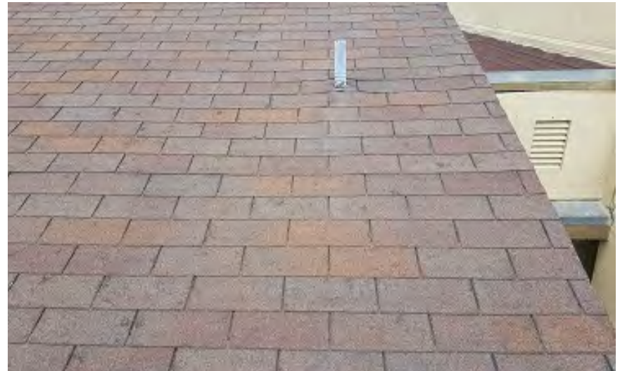
Photo 72 – West Building Roof showing Hail Damage (Looking West)
