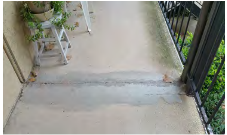
Photo 31 – 2 nd Floor: Walkway Crack
