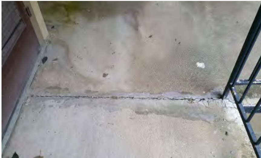
Photo 36 – 2 nd Floor: Walkway Crack
