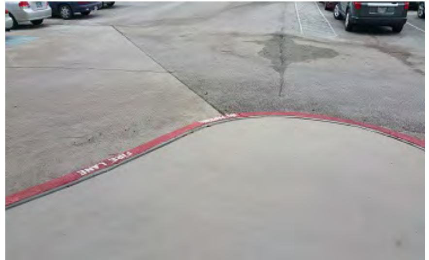
Photo 63 – North Parking Lot: Deteriorated Concrete Joints
