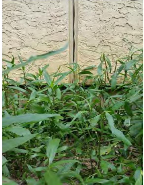
Photo 50 – West Building: Deteriorated South Expansion Joint at Base
