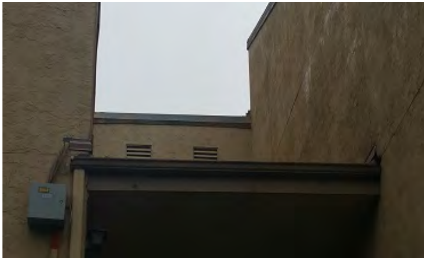
Photo 71 – 3 rd Floor Deteriorated Walkway Canopy Façade between North and West Buildings
