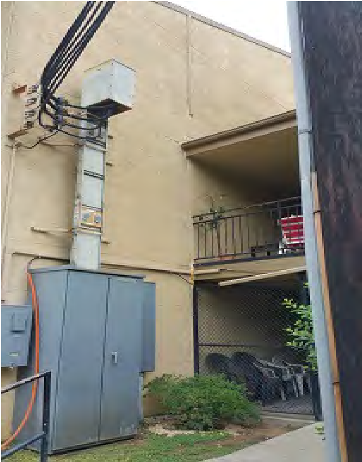
Photo 60 – East Building: North Facade
