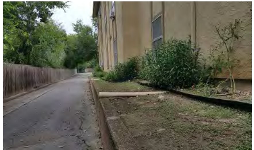
Photo 53 – West Building: Improper Drainage (Looking North)
