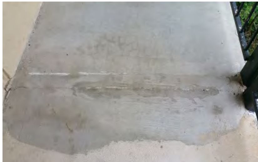
Photo 46 – 3 rd Floor: Walkway Crack
