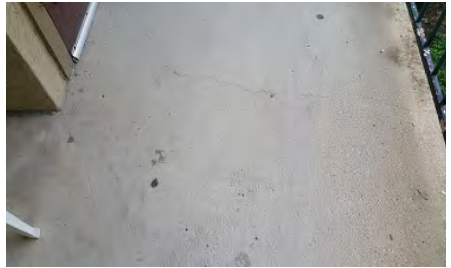
Photo 33 – 2 nd Floor: Walkway Crack
