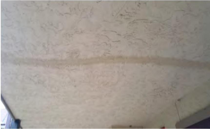
Photo 30 – 2 nd Floor: Walkway Ceiling Crack
