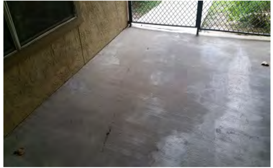
Photo 20 – Walkway Crack near NE Community Exit
