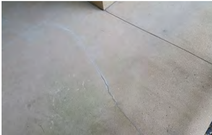
Photo 29 – 2 nd Floor: Walkway Crack
