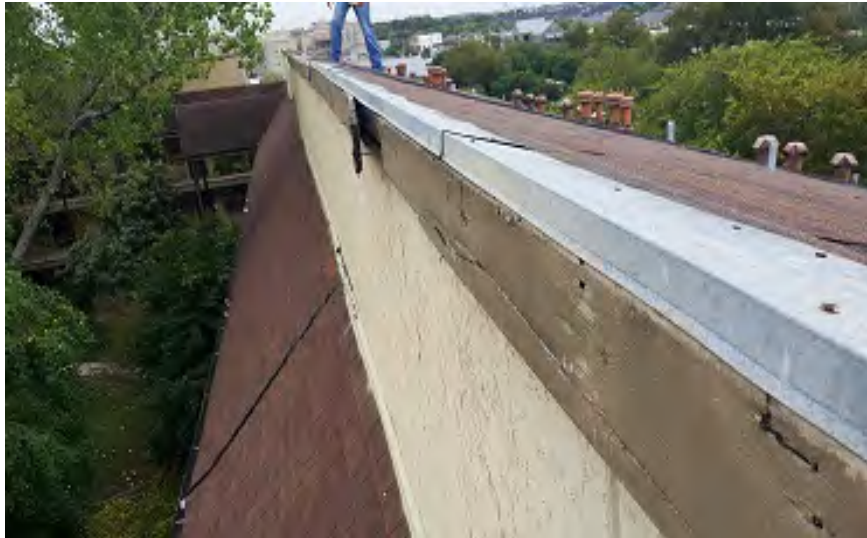
Photo 93 – West Building: Deteriorated Ridge Flashing and Canopy Roof (Looking South)
