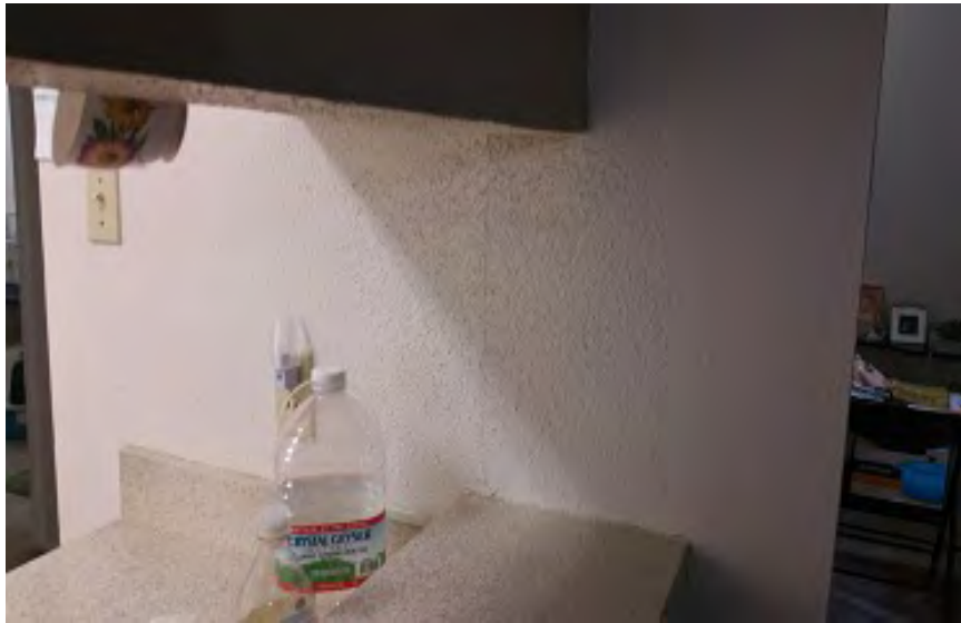
Photo 5 – Unit 113: Cracks at Kitchen Counter
