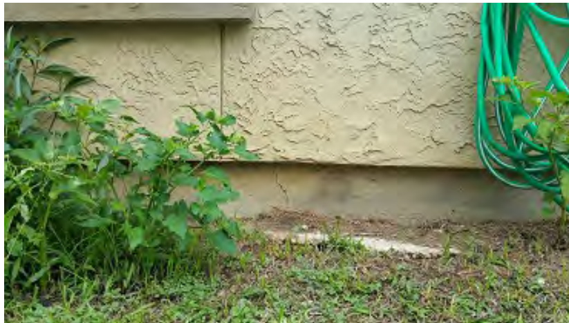
Photo 51 – West Building Foundation Crack
