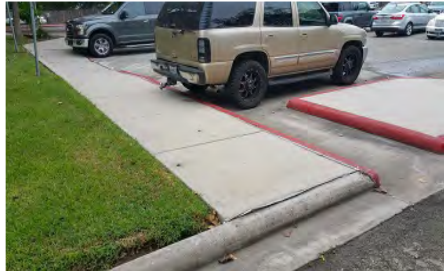
Photo 62 –North Parking Lot: Deteriorated Concrete Joints
