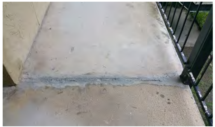
Photo 37 – 2 nd Floor: Walkway Crack
