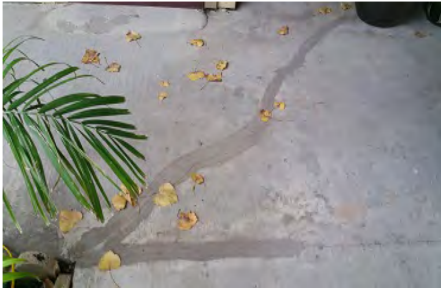
Photo 1 – Walkway Cracks near Unit 113
