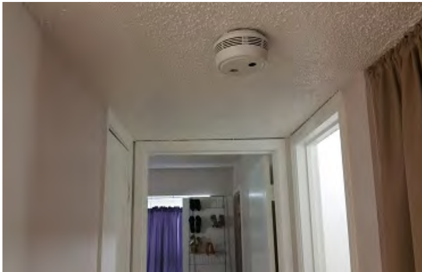
Photo 7 – Unit 113: Cracks above doors in Hallway
