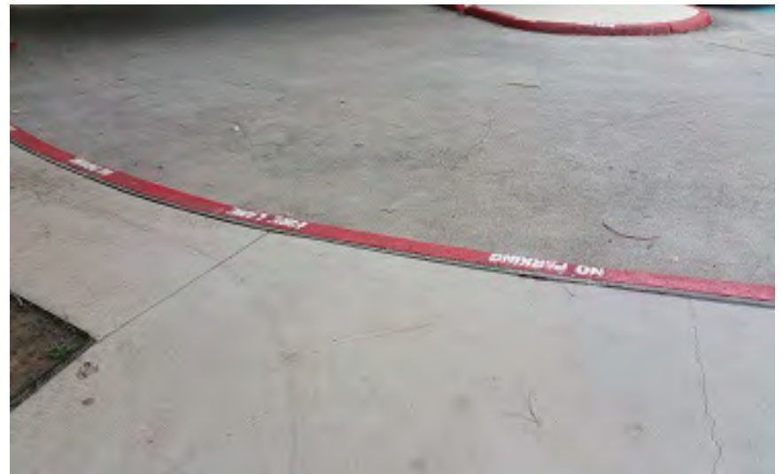
Photo 64 –North Parking Lot: Deteriorated Concrete Joints
