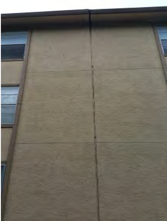
Photo 56 – East Building: Deteriorated South Expansion Joint
