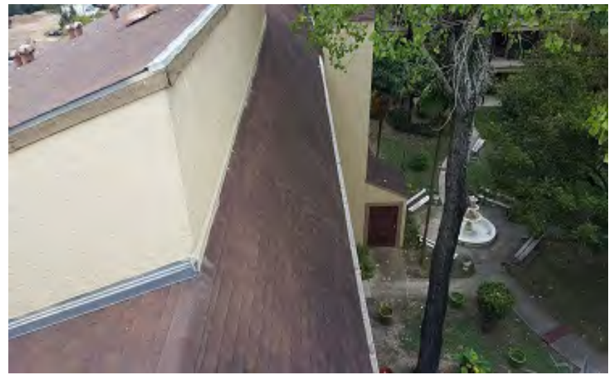
Photo 82 – South Building Walkway Canopy Roof showing Hail Damage and deteriorated Ridge Construction (Looking West)
