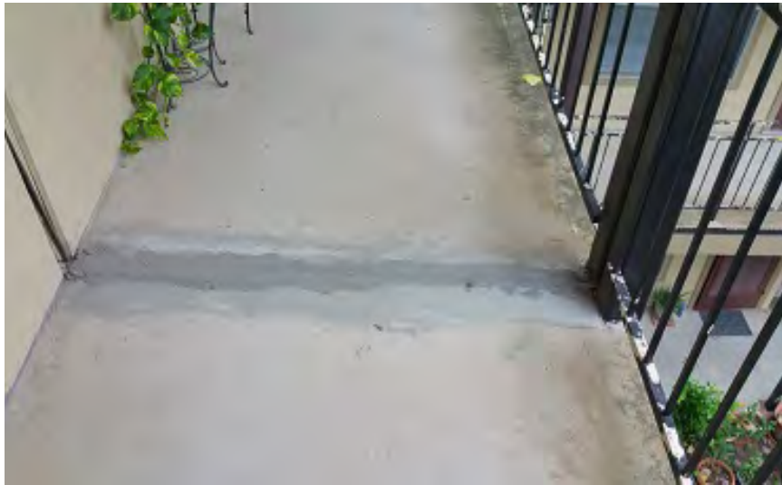
Photo 38 – 3 rd Floor: Walkway Crack
