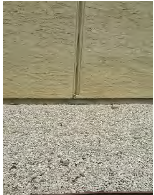
Photo 59 - East Building: Deteriorated North Expansion Joint at Base
