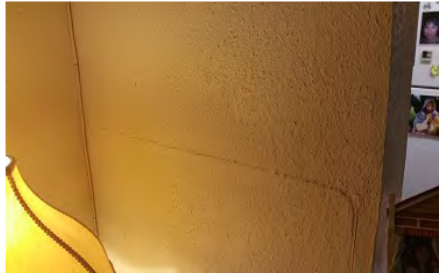
Photo 17 – Unit 108: Wall Crack in Living Room
