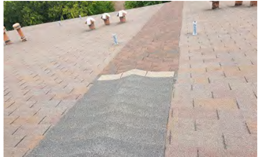
Photo 78 – East Building Southern Roof Expansion Joint Improperly Covered with a Shingle Patch
