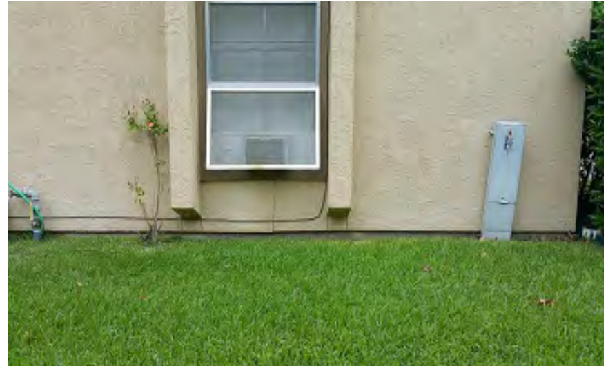
Photo 61 – North Building: East Façade with Crack below Window
