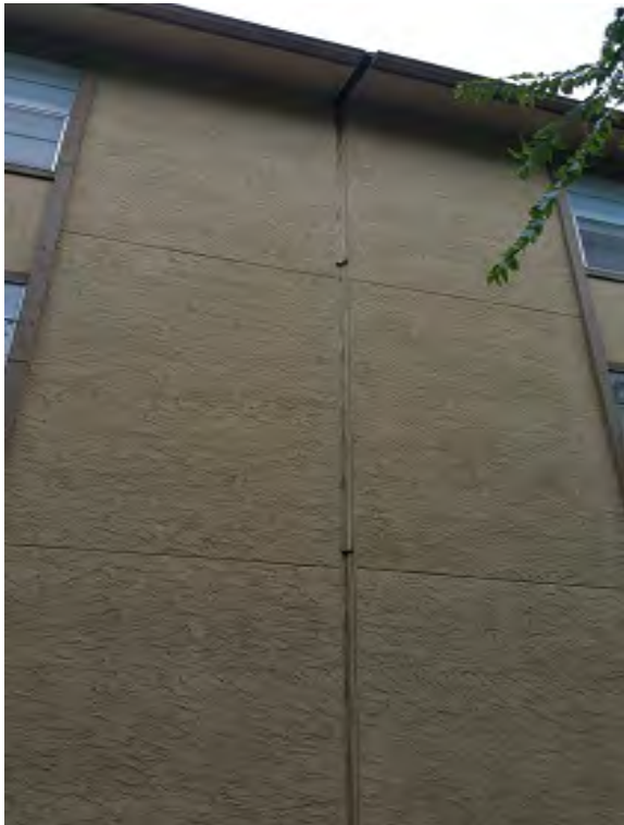
Photo 58 - East Building: Deteriorated North Expansion Joint
