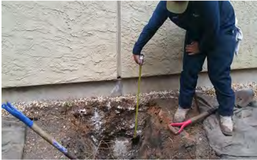
Photo 69 – East Building: Test Pit 2
