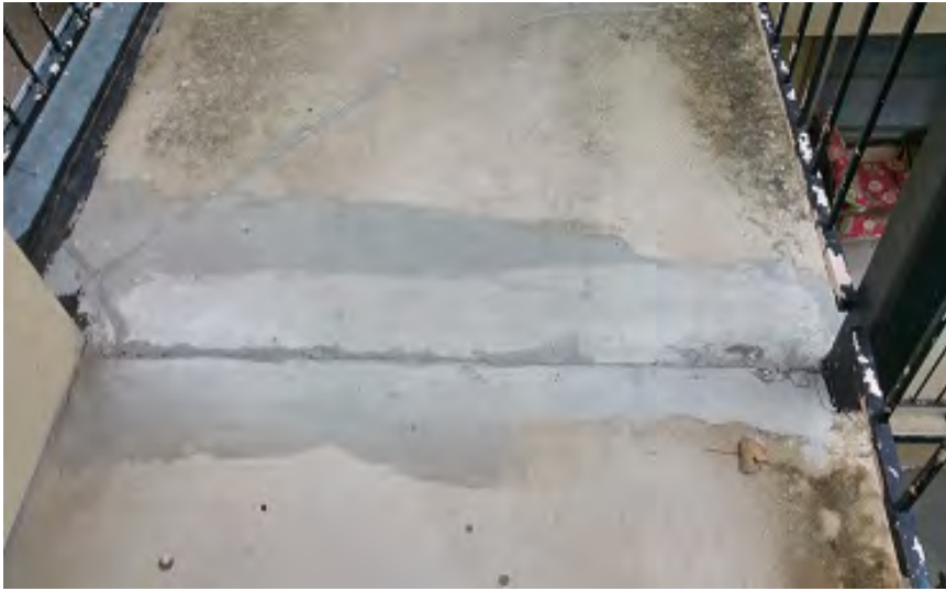
Photo 42 – 3 rd Floor: Walkway Crack
