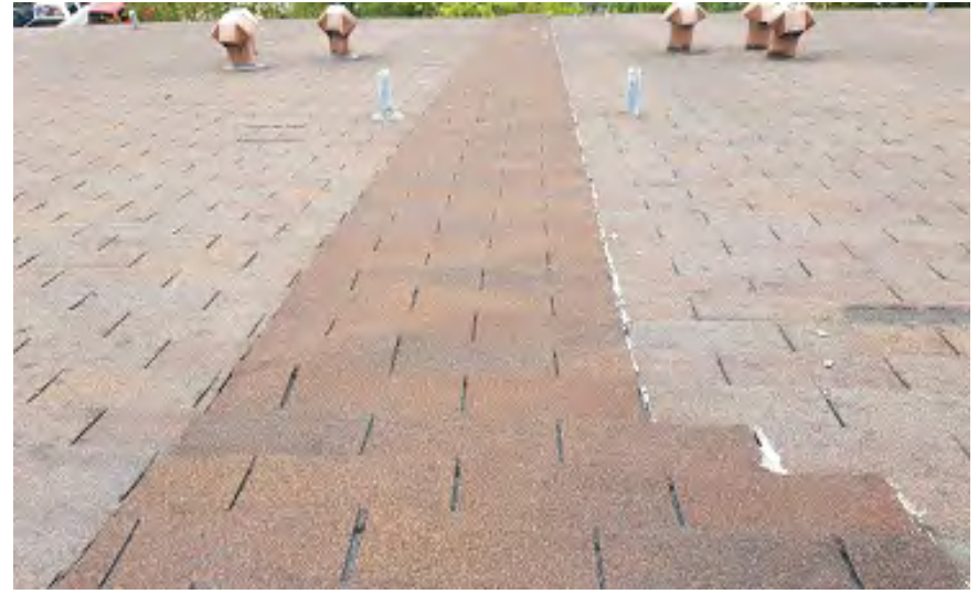
Photo 90 – West Building Southern Roof Expansion Joint Improperly Covered with a Shingle Patch
