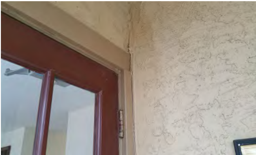
Photo 44 – 3 rd Floor: Crack at Door Frame near Elevator Lobby
