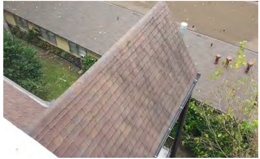
Photo 74 – East Building: North Stairway Roof showing Hail Damage
