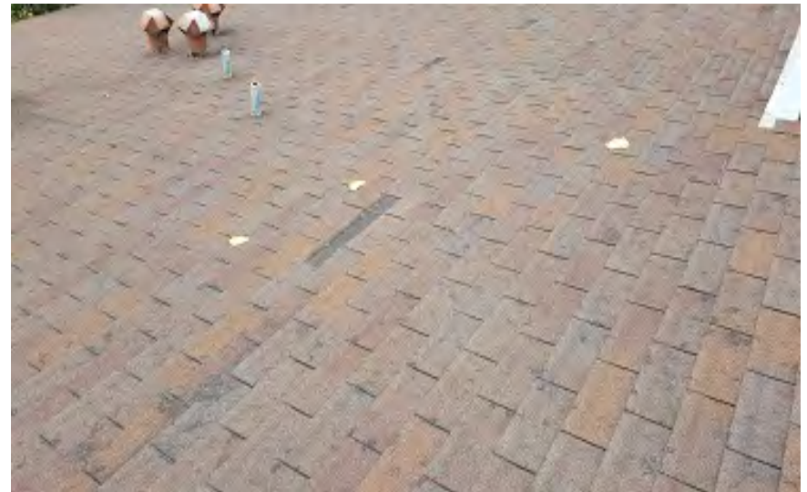
Photo 86 – West Building Roof showing Hail Damage (Looking North)
