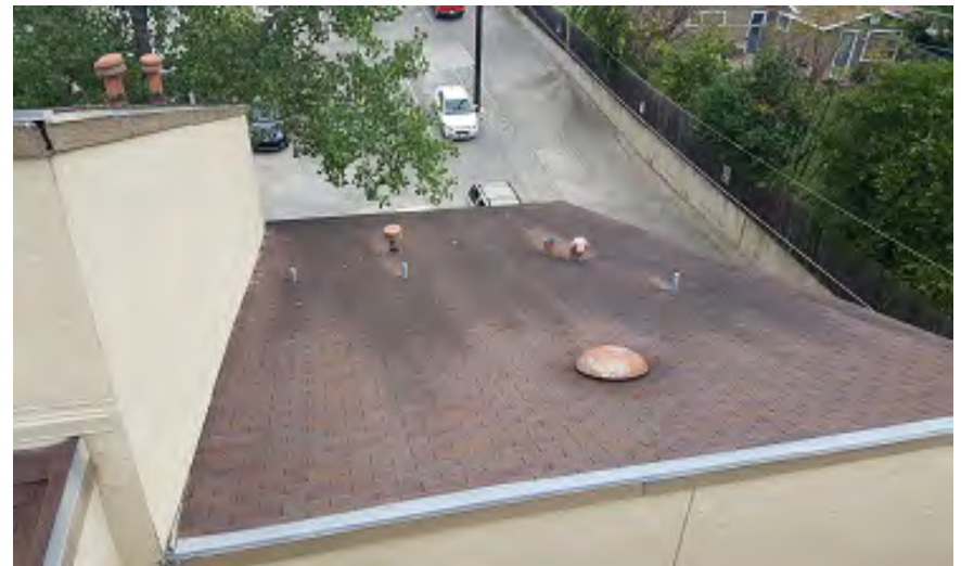
Photo 96 – North Building: East End showing Deteriorated Ridge and Rake Flashing and Facade Cracks (Looking North)
