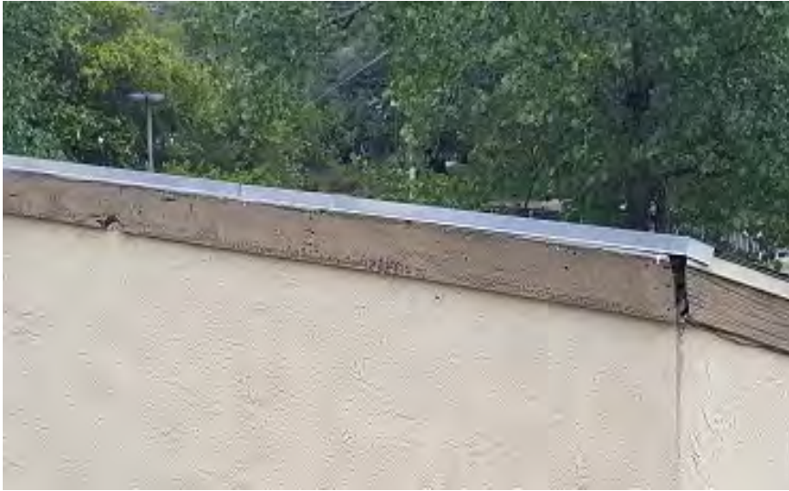
Photo 97 – North Building: Deteriorated Ridge and Rake Flashing
