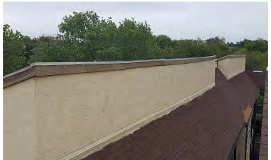
Photo 84 – North Building: Walkway Canopy Roof (Looking East)
