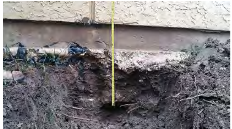
Photo 68 –West Building: Test Pit 1
