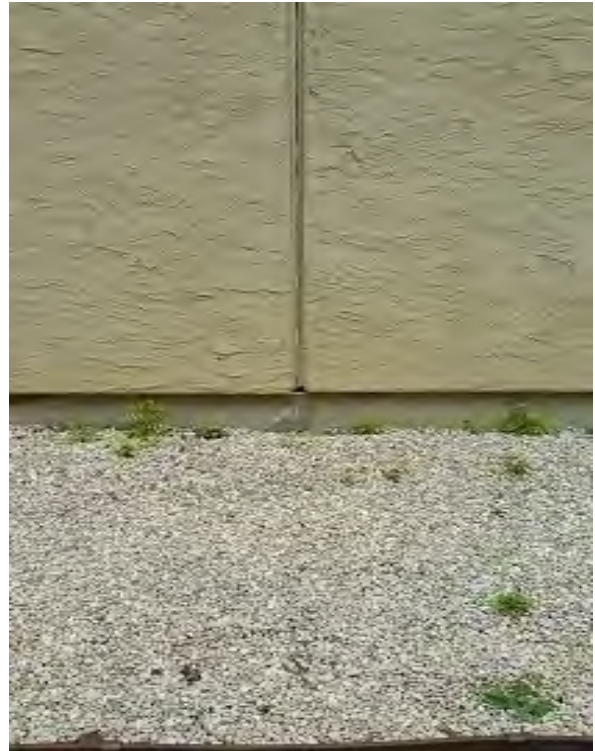
Photo 57 – East Building: Deteriorated South Expansion Joint at Base
