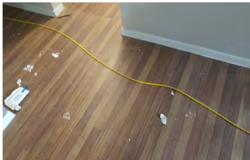
Photo 10 – Unit 112: Heaving of Floor near Kitchen
