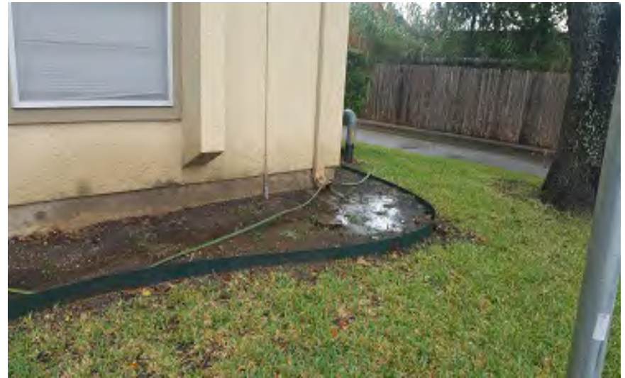
Photo 67 – North Building: Improper Drainage at NW Corner
