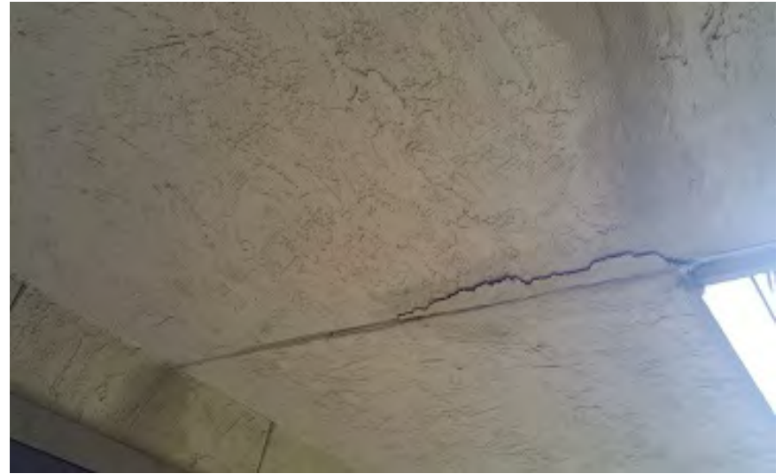
Photo 24 – Walkway Ceiling Crack near Unit 132
