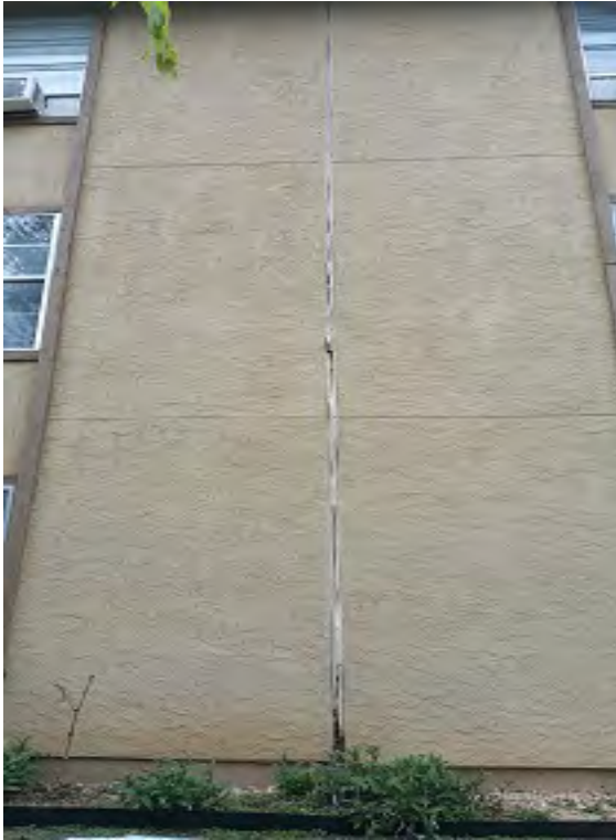
Photo 47 – West Building: Deteriorated North Expansion Joint
