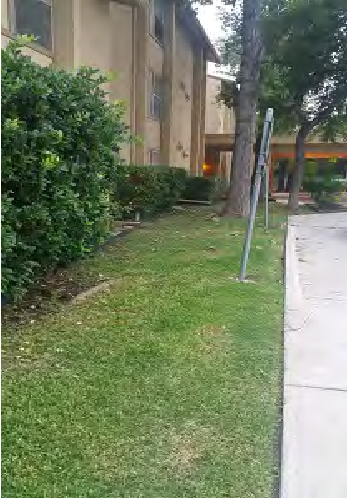
Photo 66 – North Building: Improper Drainage back towards Building (Looking West)
