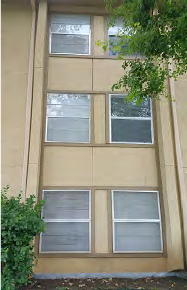
Photo 65 – North Building: North Façade Window Area with Vertical Crack and Sheetmetal Dam at Base
