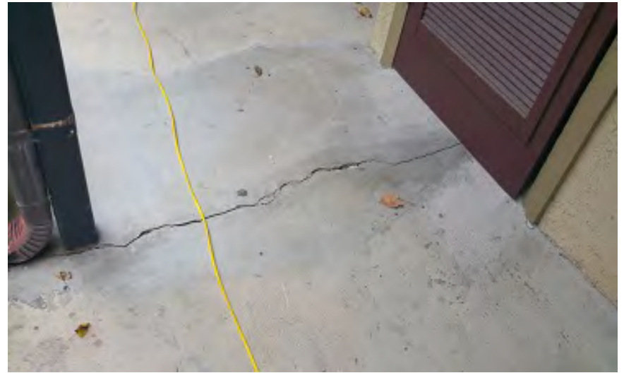
Photo 22 – Walkway Crack near Unit 102
