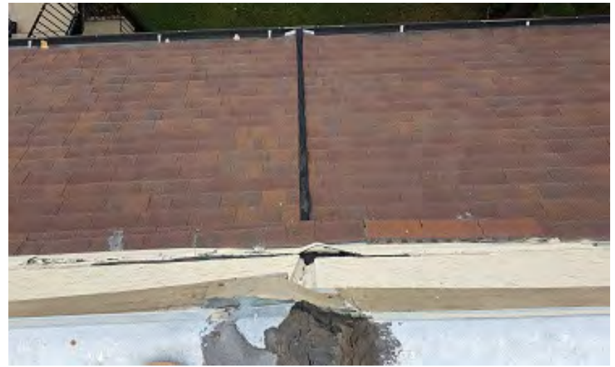
Photo 92 – West Building: Southern Deteriorated Expansion Joint at Walkway Canopy Roof
