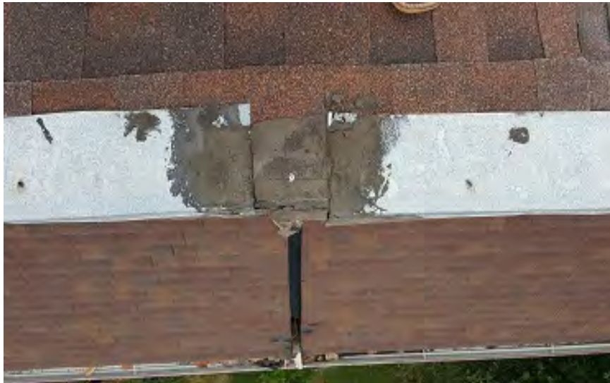
Photo 77 – East Building: Northern Deteriorated Expansion Joint at Walkway Canopy Roof
