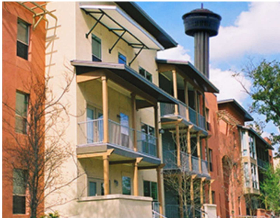
REFUGIO PLACE APARTMENT HOMES
