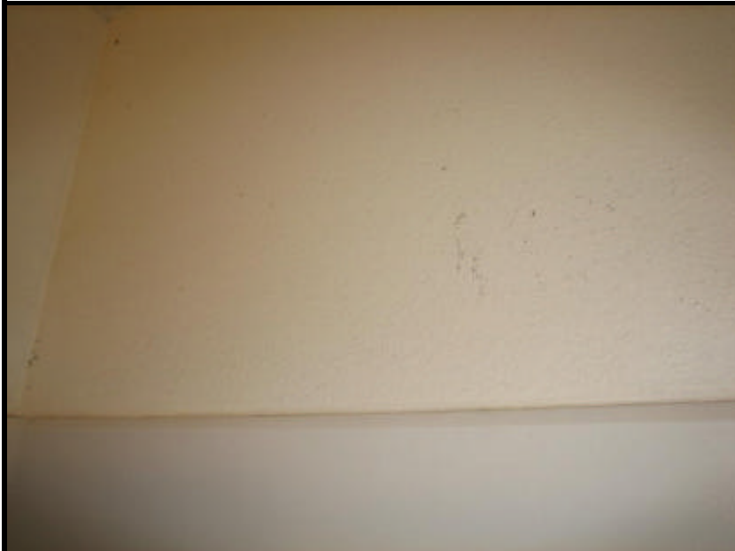
View of area above main bathroom
