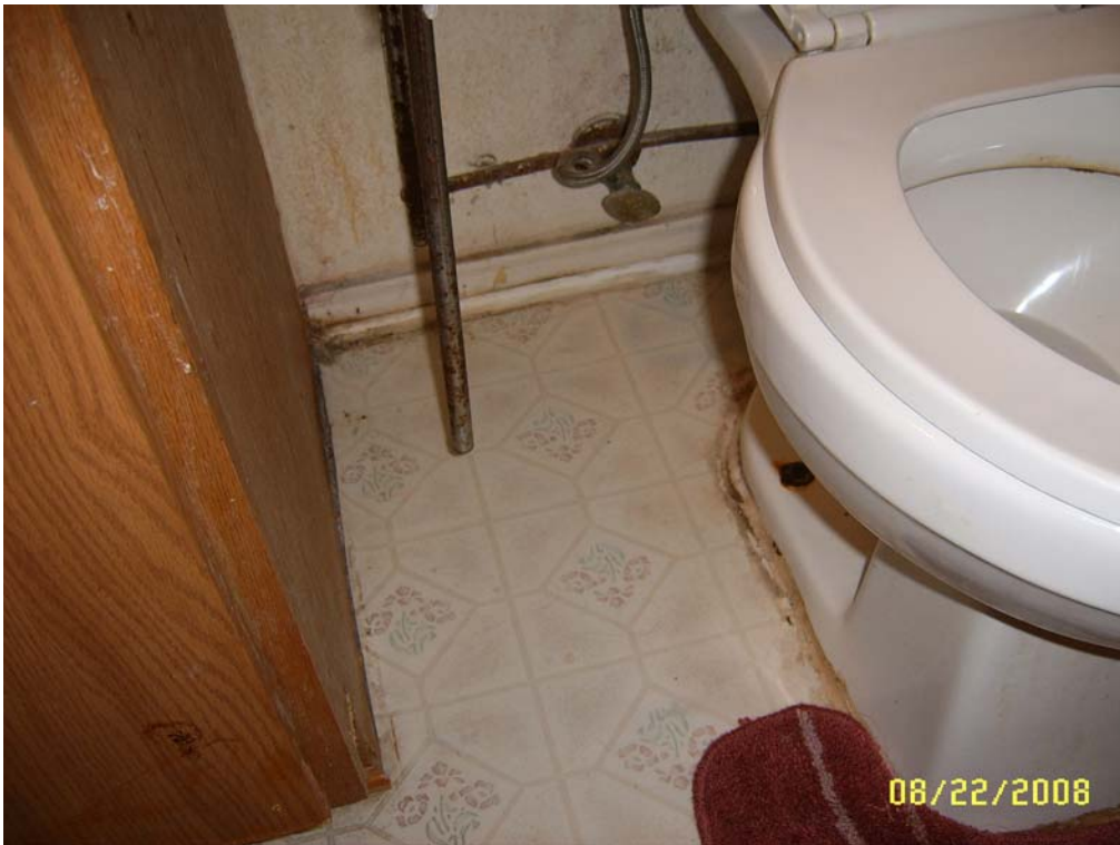
Master Bath – toilet area
