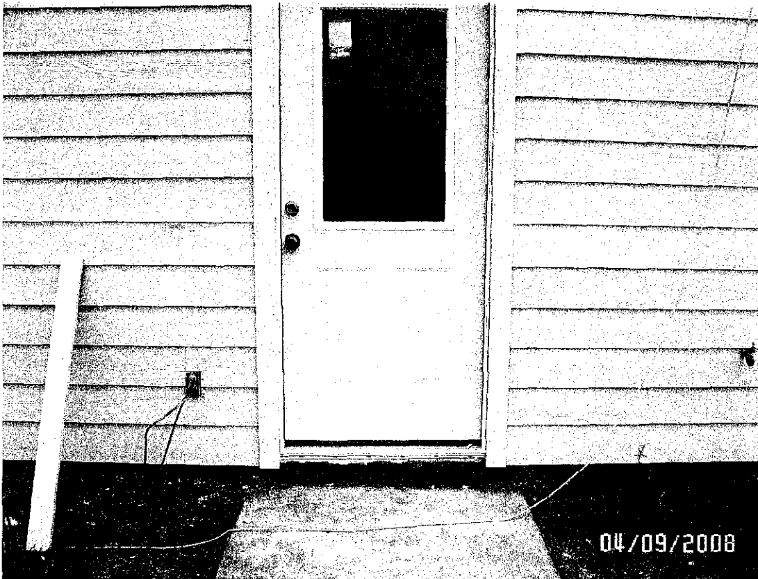
New back door, frame & siding
