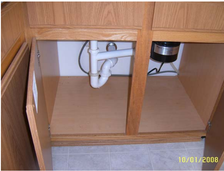
Kitchen sink area
