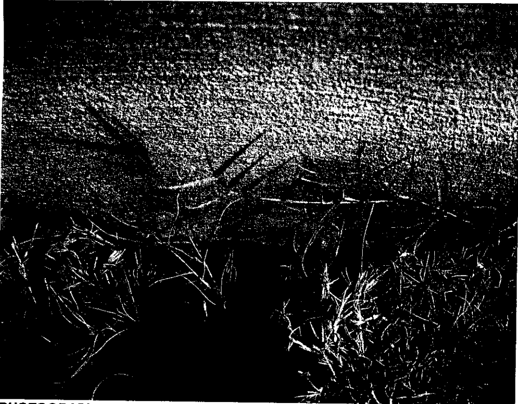
PHOTOGRAPH 7 CLOSE-UP VIEW OF DRYING SOIL CONDITIONS ALONG THE PERIMETER GRADE BEAM LOCATED ALONG THE RIGHT SIDE OF THE HOME.
