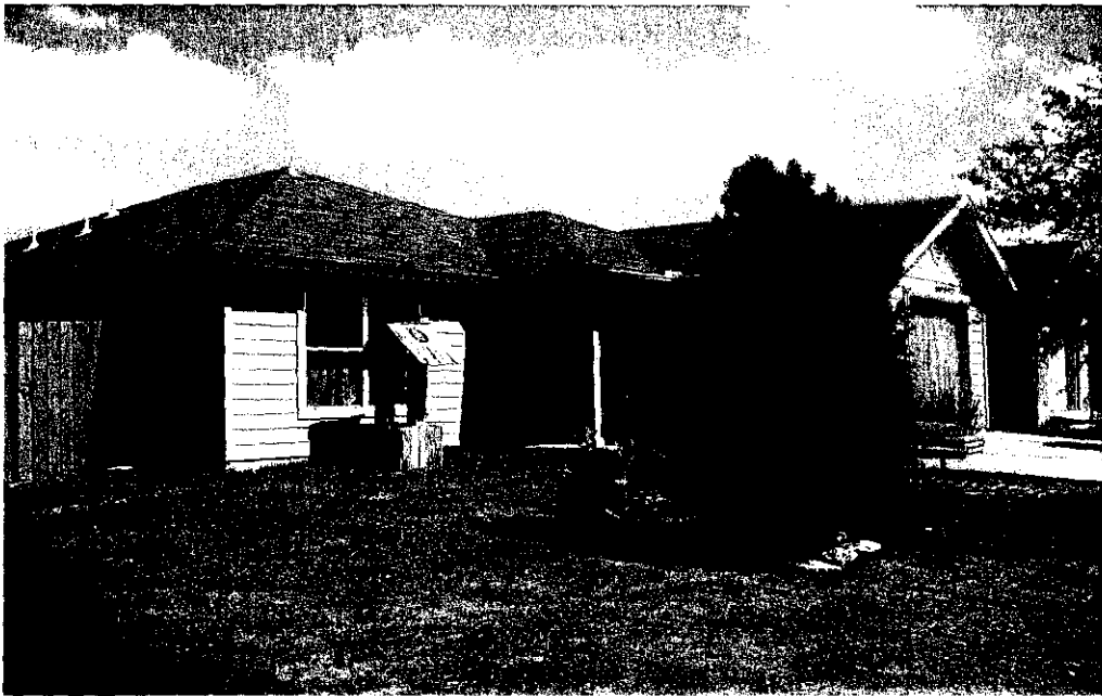
PHOTOGRAPH 2 GENERAL VIEW OF THE RIGHT FRONT CORNER OF THE HOME.
