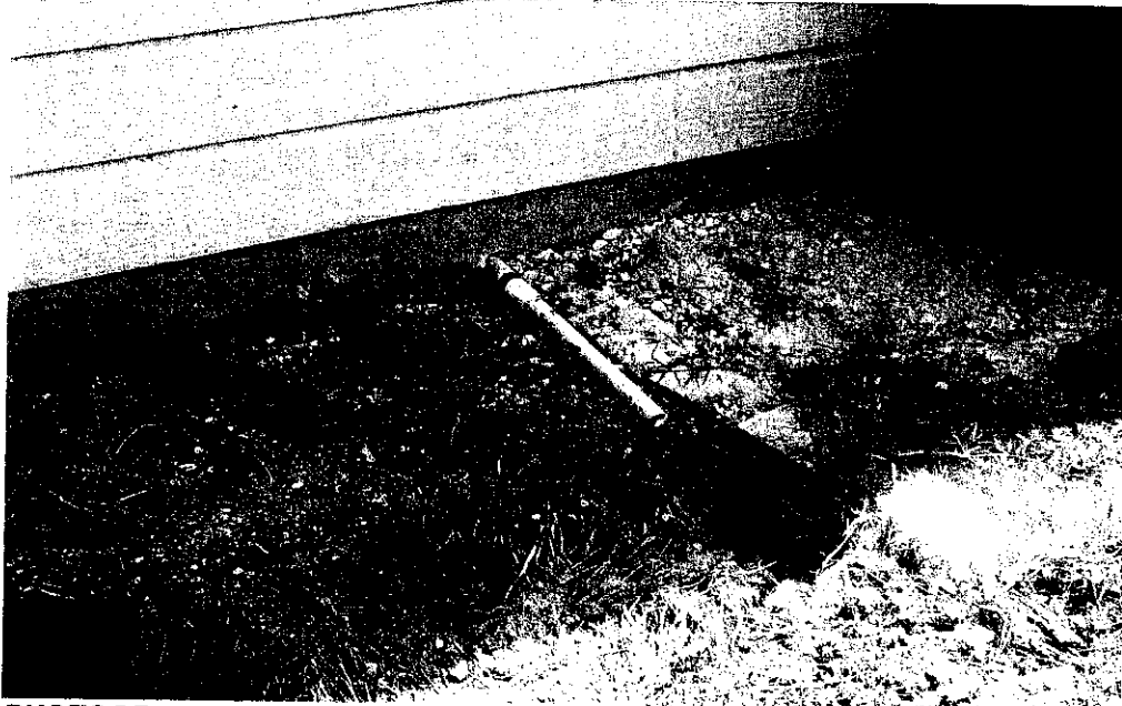
PHOTOGRAPH 8 GENERAL VIEW OF THE CONDENSATE DRAIN LINE AND T/P R DRAIN PIPING LOCATED AT THE PERIMETER GRADE BEAM ALONG THE LEFT SIDE OF THE HOME.
