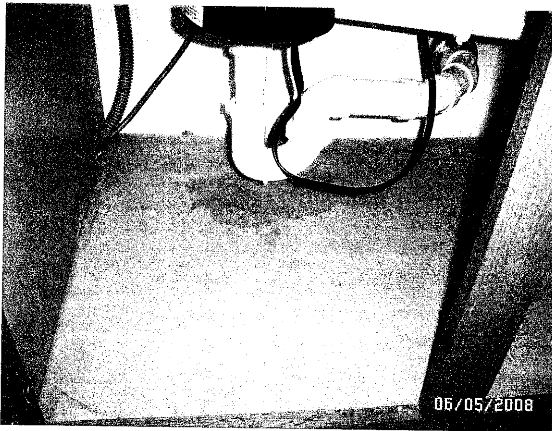
water spots below kitchen sink
