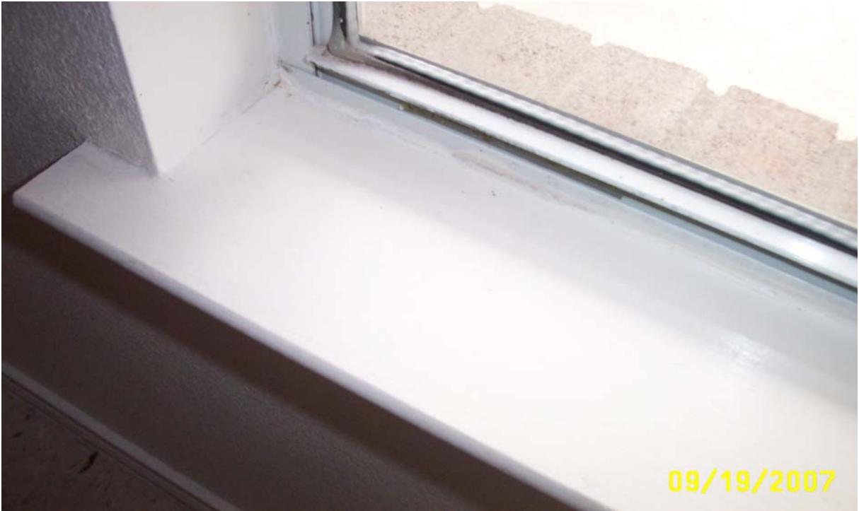
Photo 1: Kitchen- Clean exterior window.
