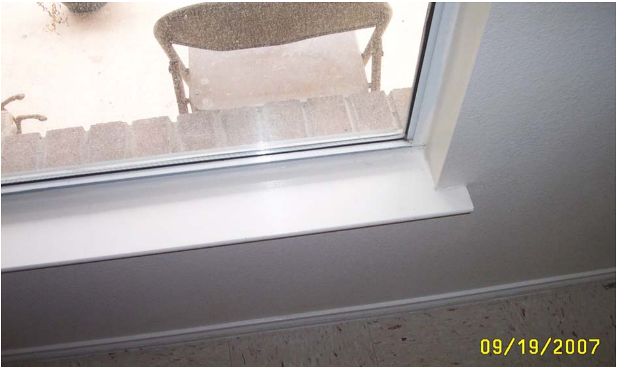
Photo 2: Kitchen- Clean exterior window.
