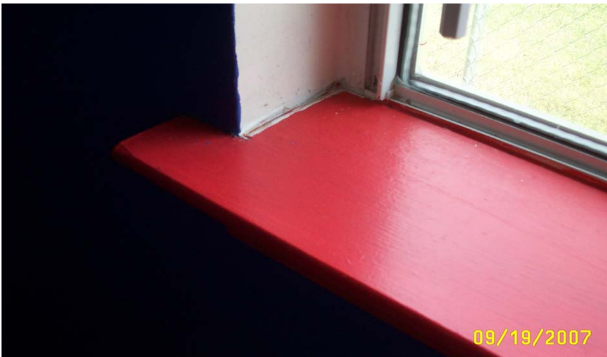
Photo 8: Bedroom #3- Removed caulk along exterior wall window.
