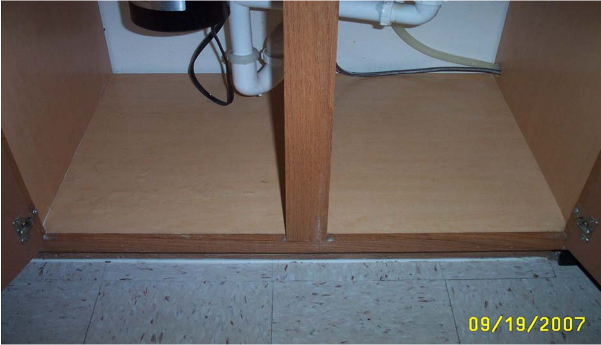
Photo 3: Kitchen- Clean shelf below sink.
