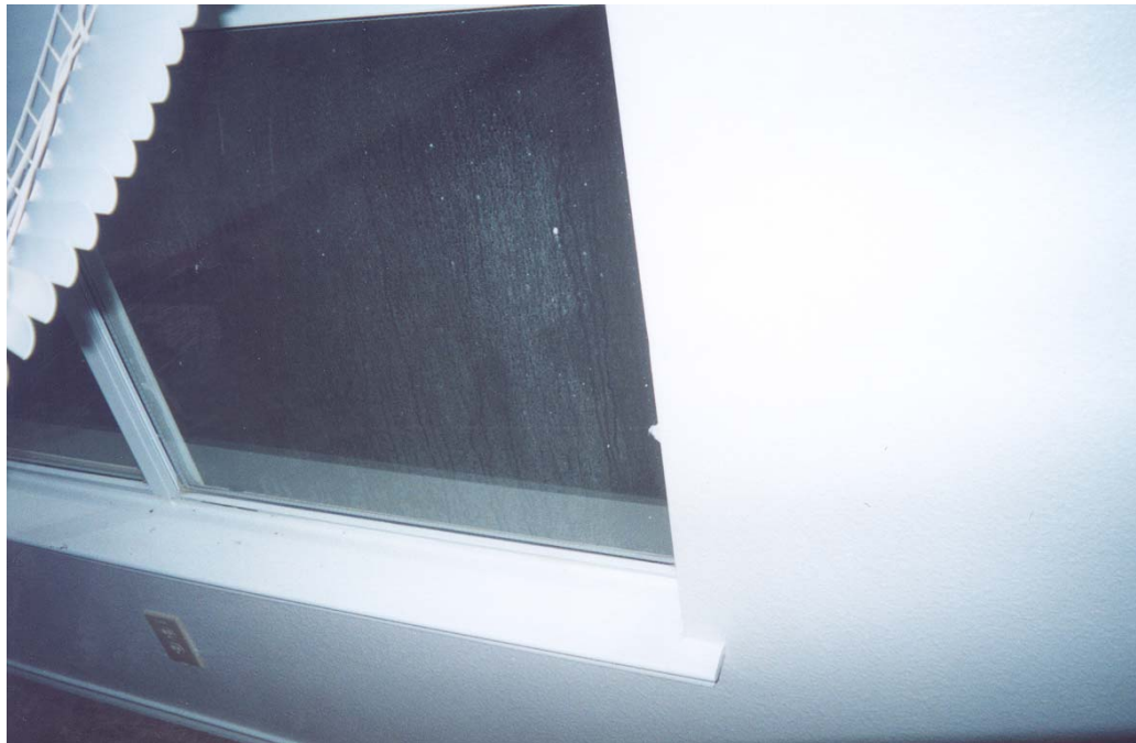
PHOTO 8: View of typical clean window sills.
