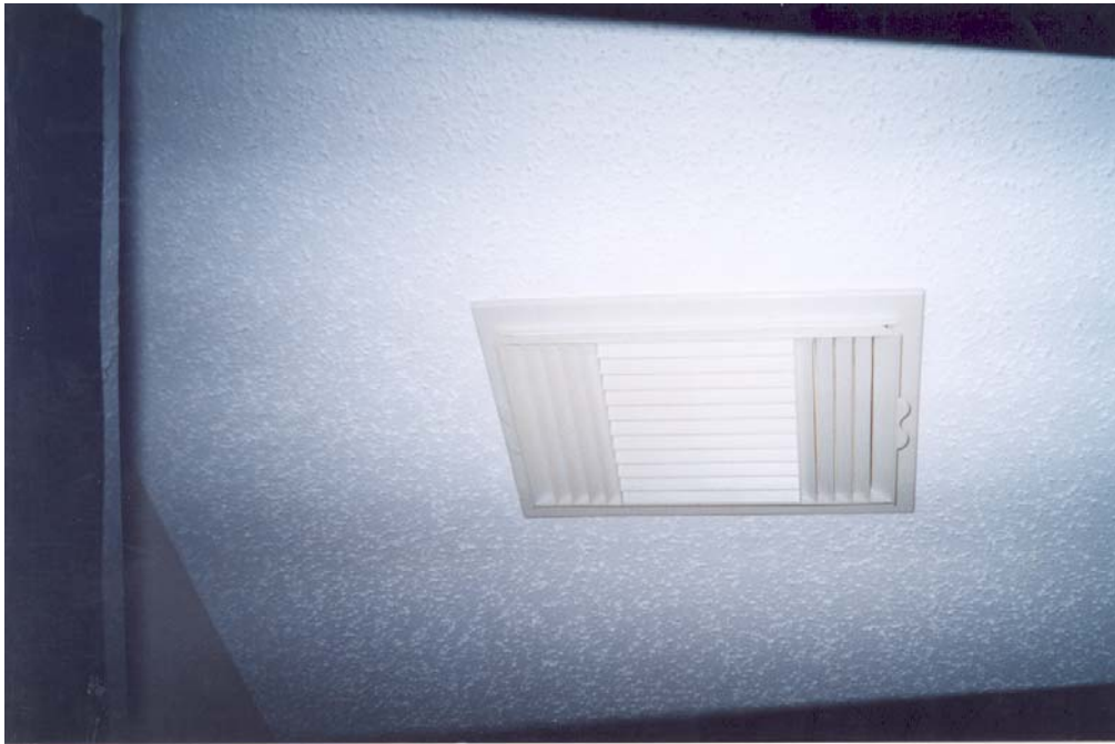
PHOTO 3: Additional view of a clean HVAC outlet.
