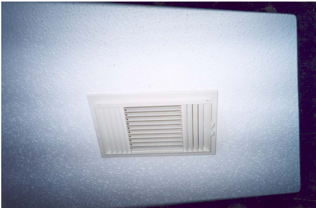
PHOTO 4: Additional view of a clean HVAC outlet.
