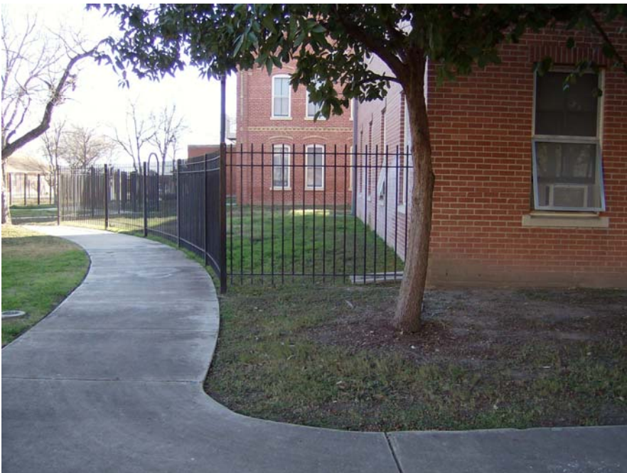
Attach new fencing to existing fence (no gaps)
