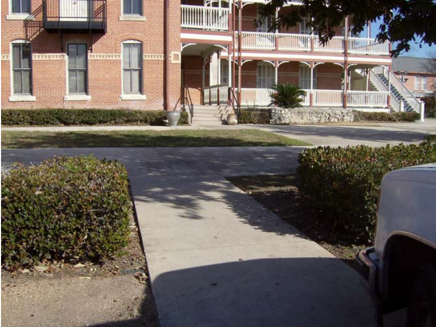
Gate install here by The Convent; second gate at sidewalk between the hedges and B Building.
